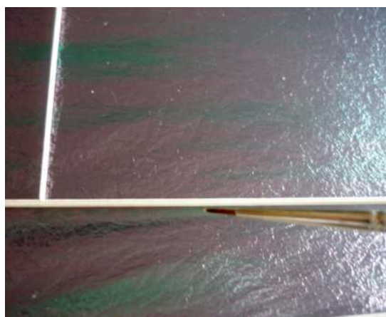
Thin adhesive applied to edges
